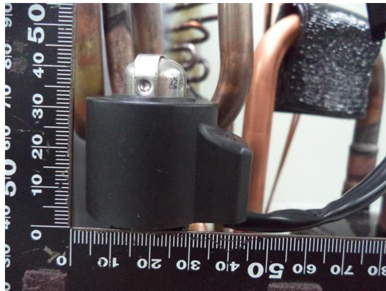
257. RAV-GP801AT-E, RAV-GP801ATJ-E, RAV-GP801AT-TR, PMV Coil
