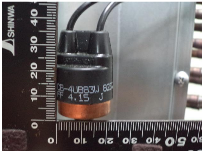
259. RAV-GP801AT-E, RAV-GP801ATJ-E, RAV-GP801AT-TR, Pressure switch
