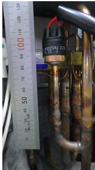
155. RAV-GP561ATP-E, RAV-GP561ATJP-E, RAV-GP561ATP-TR, Pressure Switch
