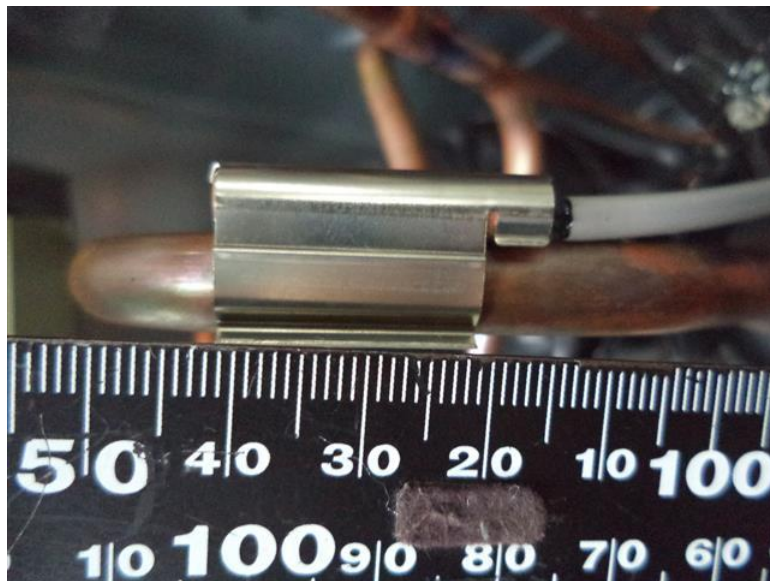
81. RAV-GM401ATP-E, RAV-GM401ATJP-E, RAV-GM401ATP-TR, Thermistor
