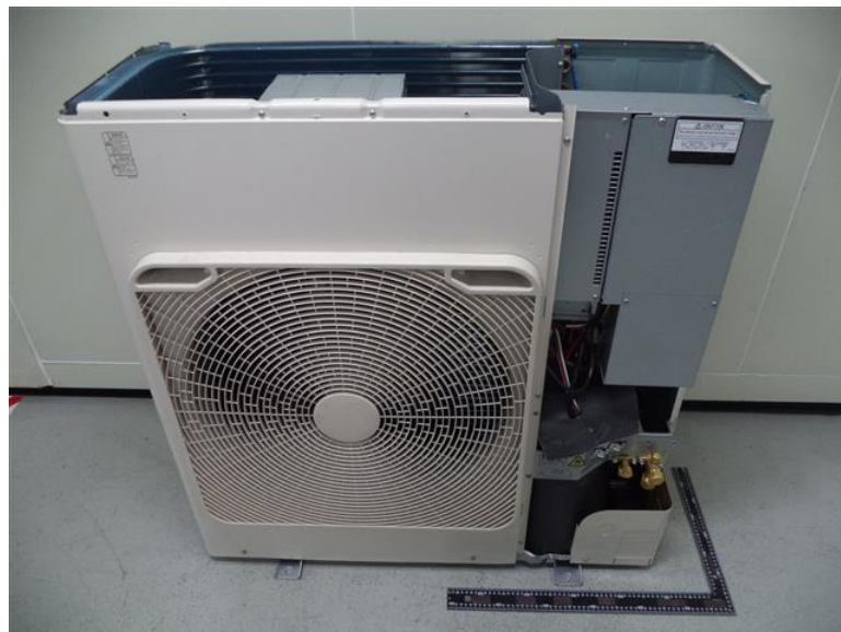
243. RAV-GP801AT-E, RAV-GP801ATJ-E, RAV-GP801AT-TR, Internal construction
